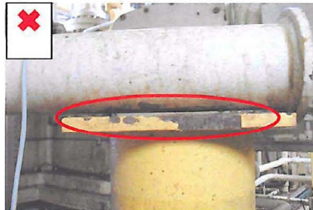
Pipework clear of resting support (air gap)
