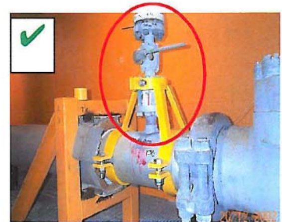
Good support of cantilevered mass
