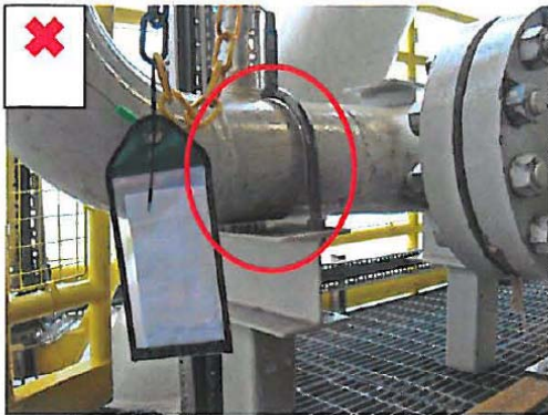
U-Bolt providing little or no restraint to vibration; no lining between U-Bolt and pipe
