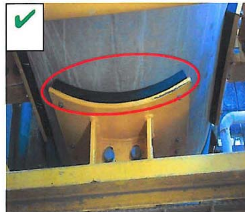
Resilient pad between support and pipe protects against fretting damage
