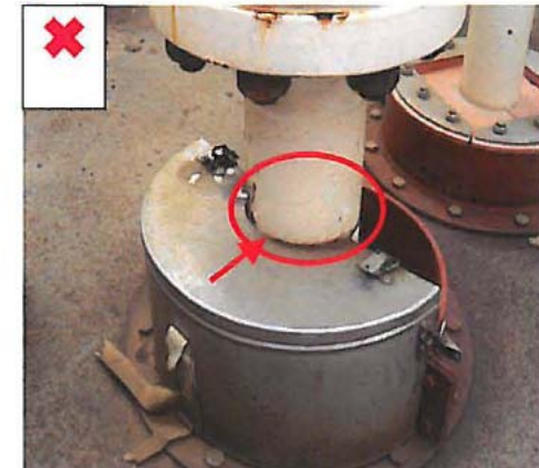
Fretting damage to pipe caused by pipework vibrating relative to deck penetration cover
