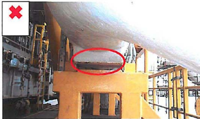
U-Bolt providing little or no restraint to vibration; no lining between U-Bolt and pipe
